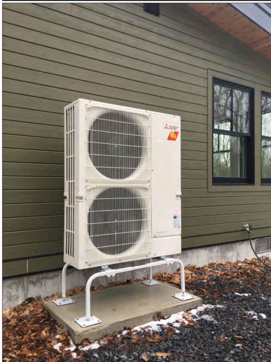
A Mitsubishi air source heat pump (mini split).
